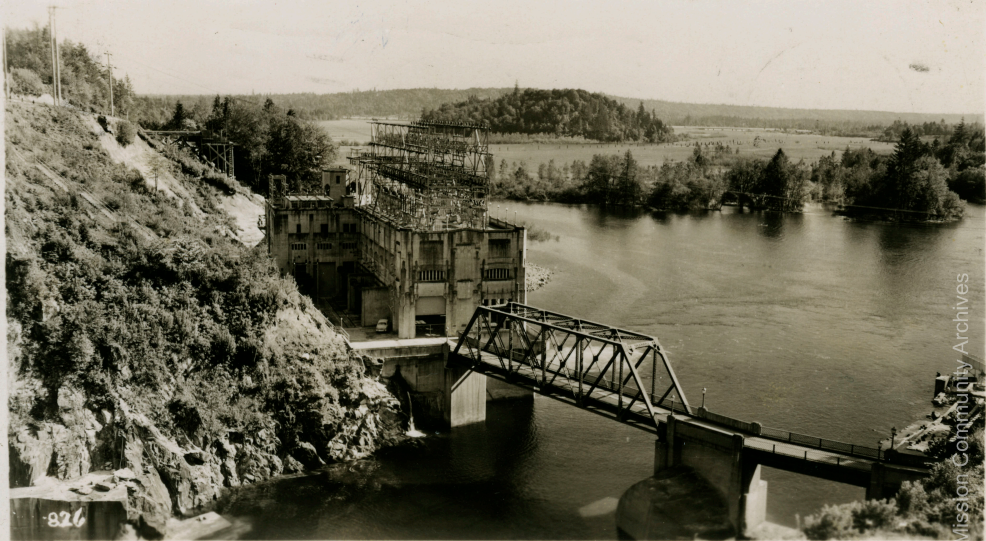
Ruskin Power Plant, near Mission City, B. C.
